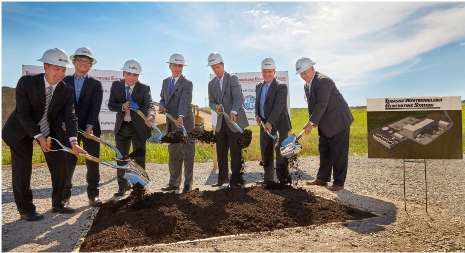
Ground is ceremonially broken at the Tenaska Westmoreland Generating Station project near Smithton in Westmoreland County on Aug. 24, 2016.
